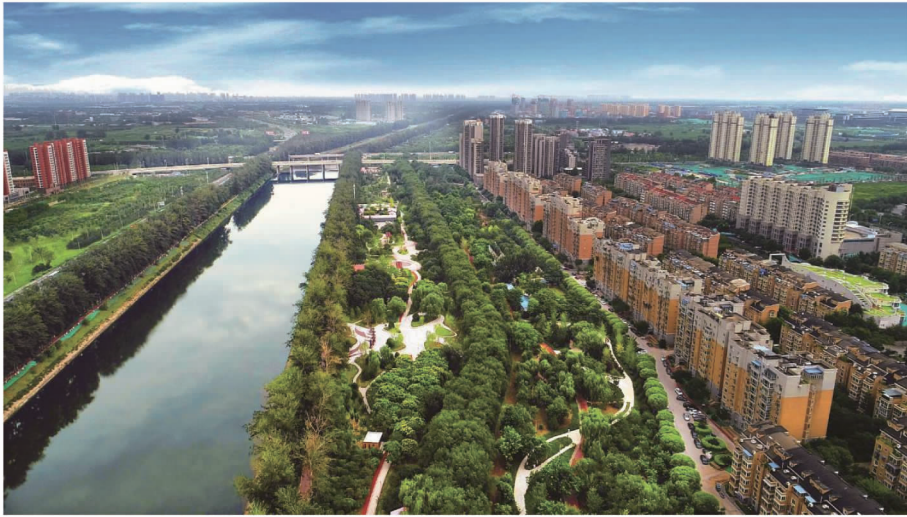
图2 减河公园鸟瞰 Fig.2 Aerial view of Jianhe Park
